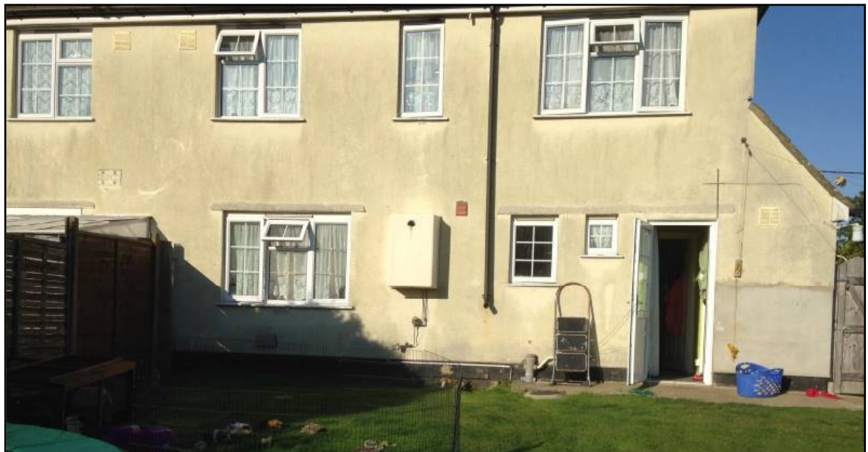
Figure 5 rear elevation from site visit
